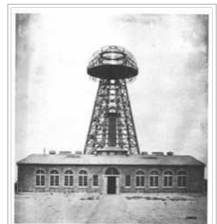
Wardenclyffe tower, a huge Tesla coil built by Tesla at Shoreham, New York, 1901-1904 as a prototype wireless power transmitter. It was never completed
