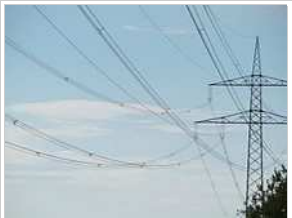
The 3-wire bundles in this power transmission installation act as a single conductor. A single wire using the same amount of metal per kilometer would have higher losses due to the skin effect.
