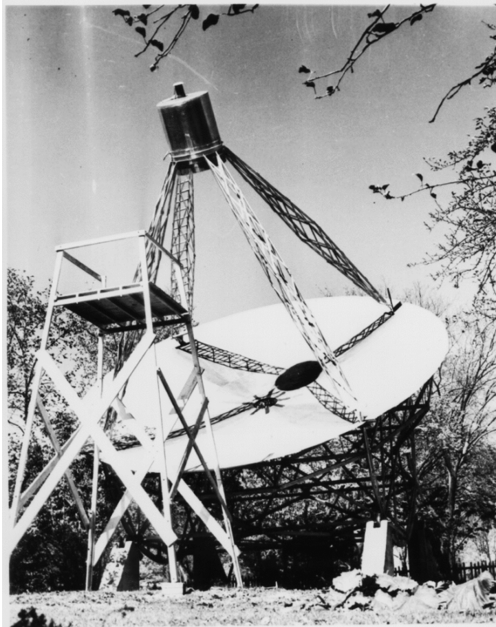
Slika 1.3: Radioteleskop: Grote Reber Wheaton, Illinois, 1937[20]
